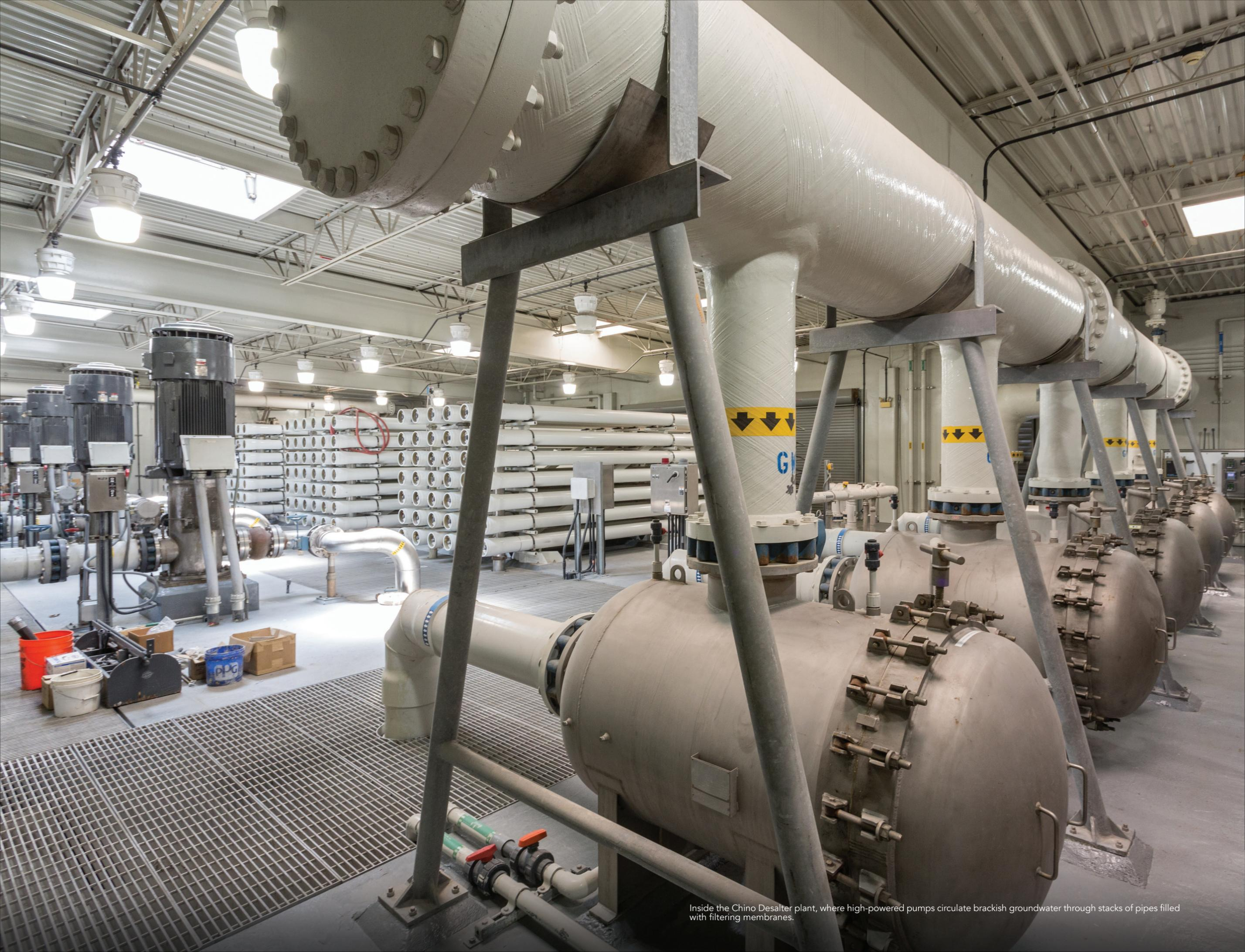
Inside the Chino Desalter plant, where high-powered pumps circulate brackish groundwater through stacks of pipes filled with filtering membranes.
