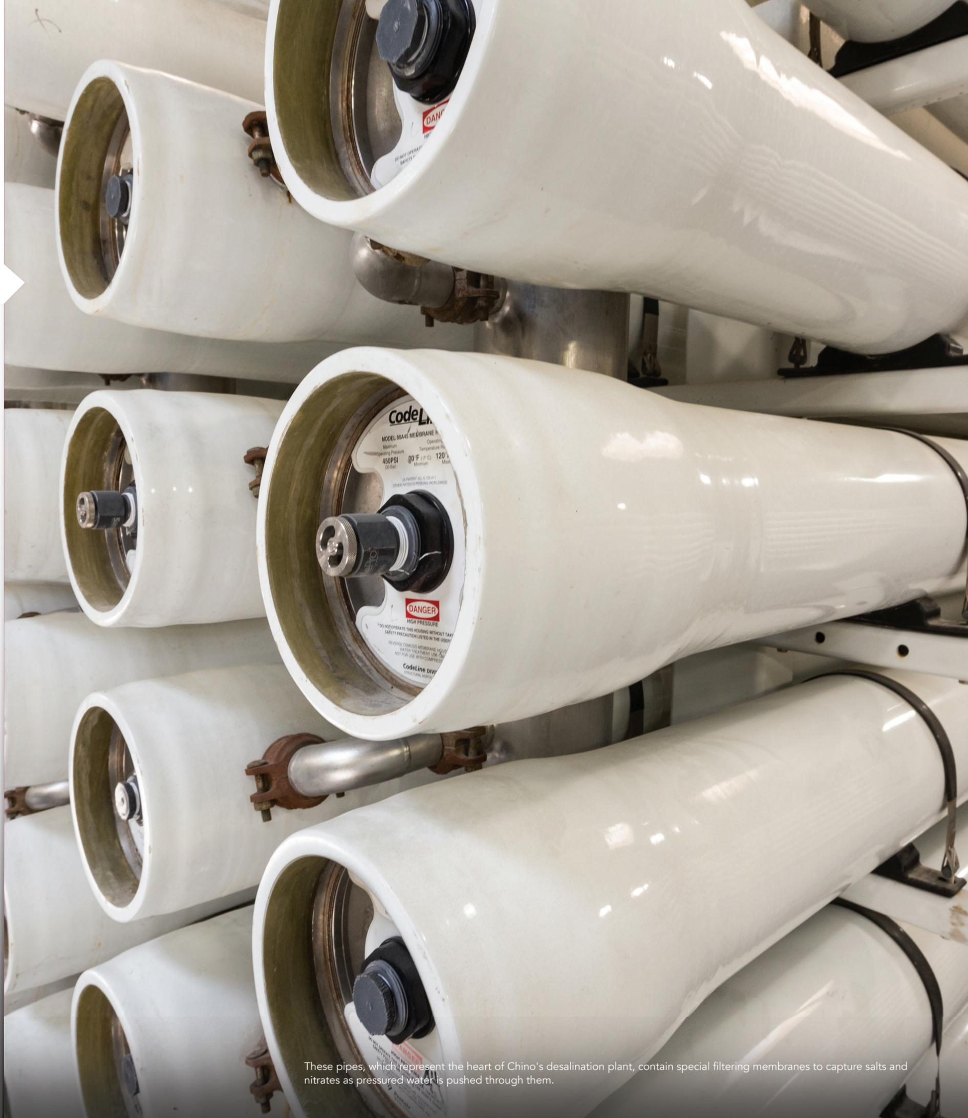
These pipes, which represent the heart of Chino's desalination plant, contain special filtering membranes to capture salts and nitrates as pressured water is pushed through them.
